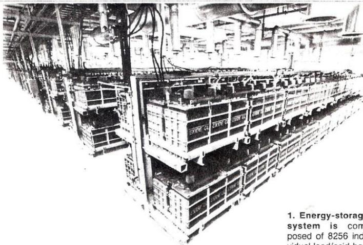
**1. Energy-storage system is composed of 8256 individual lead/acid battery cells**
