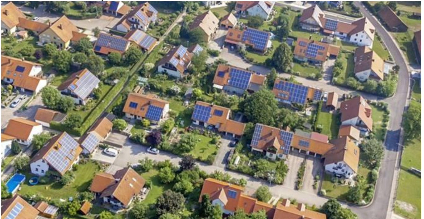
Bavarian rooftops collect the sun's energy with solar panels. Germany leads the world in installed solar capacity.
